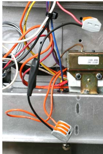
Figure 9: The new resistor is shown installed with provided connectors.
